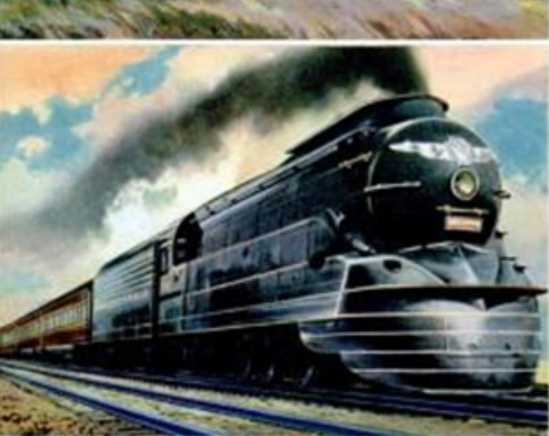
Steam power is not lagging in the railroad parade. Left, we see the Pennsylvania's "Broadway Limited," which has streamline coaches fitted with close-fitting vestibules and curving "skirt."
