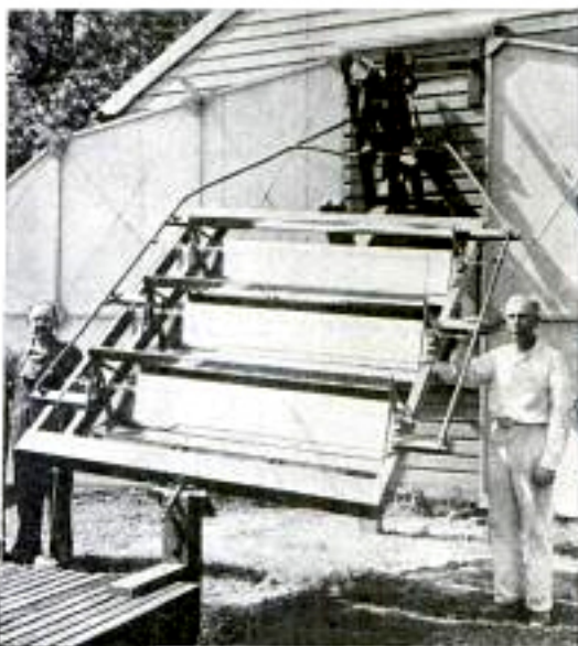
Top, aluminum mirrors focus sun's rays on tubes containing liquid which absorbs heat, flowing through pipes at side to boiler where steam is generated. Left, Dr. Abbot and aides with solar heater.
