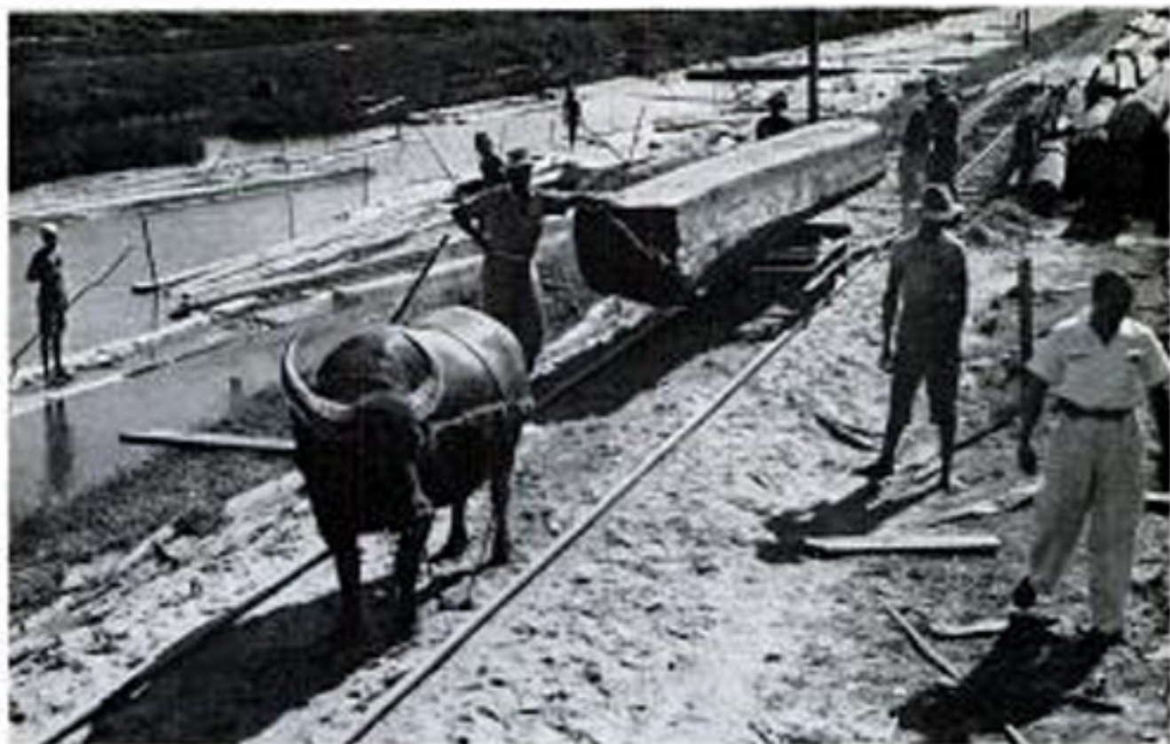
Along the canal stretches a narrow-gauge railway on which logs are hauled to the mill by water buffalo
