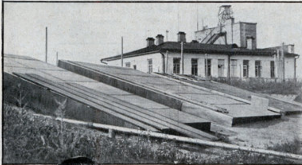
This bank of solar boilers has been installed by the Soviet Government at Tashkent in central Asia where efforts are being made to capture the sun's energy
