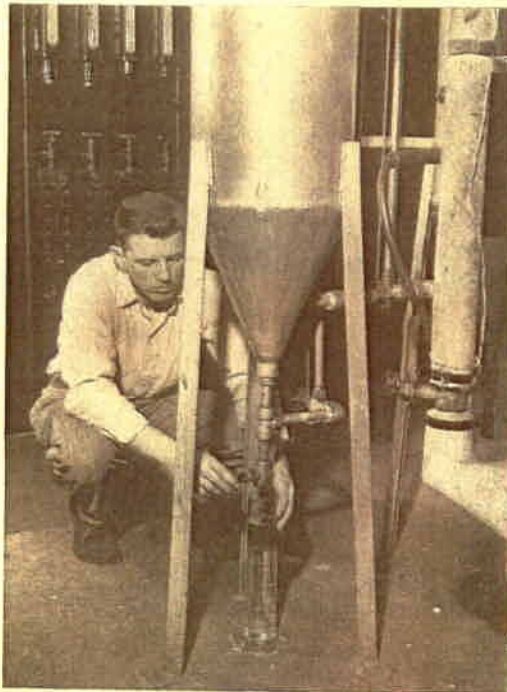
CRUDE MIXTURE of oil, water and alcohol is tapped from the tank after it is produced in synthesis towers. Standard Oil already uses similar process to make liquid fuels from natural gas at a larger pilot plant located in Louisiana.
